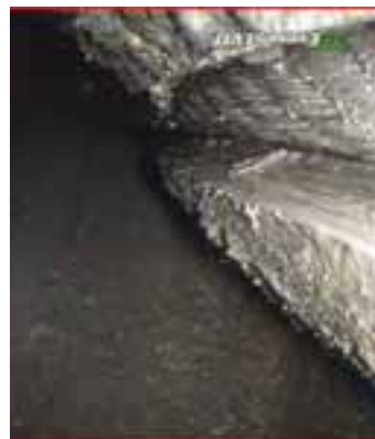
A closeup of how cable movement can create damage by rubbing by not being in alignment.
