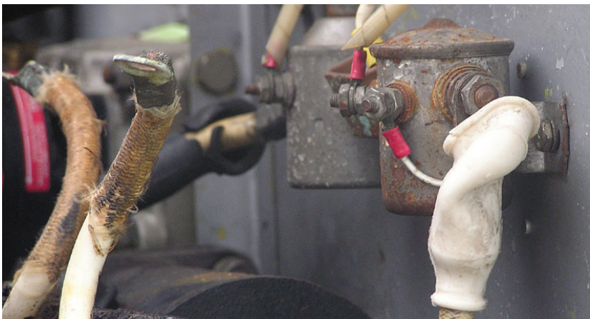
Old or neglected components and wiring are parts of an aging electrical system.
