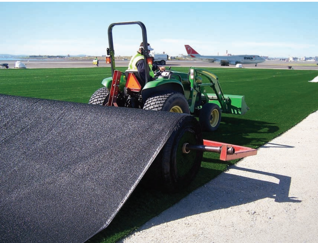
The artificial turf system allows water to drain through natural percolation and the infill provides a natural filter that can drain up to 60 gallons of water per square foot per hour. Act Global AvTurf Inc.
