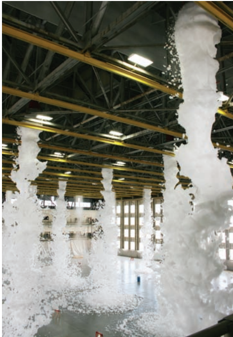
When hangar fire suppression includes deluge or high-expansion foam systems, rejecting false alarms from friendly fire is a critical function of a fire detection system. U.S. Air Force
