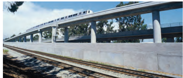
The BART to San Francisco International Airport project is a $500 million six-mile extension of underground subway, one mile of at-grade trackway and one mile of aerial bridge structure.
