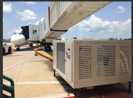
Verde 60 Ton ground mount PCA system at Sarasota International Airport
