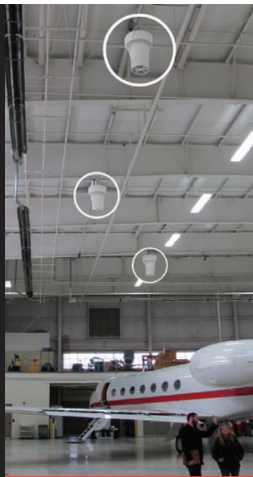
Recent Airius installation (Air Pear fans circled) in corporate jet hangar.
