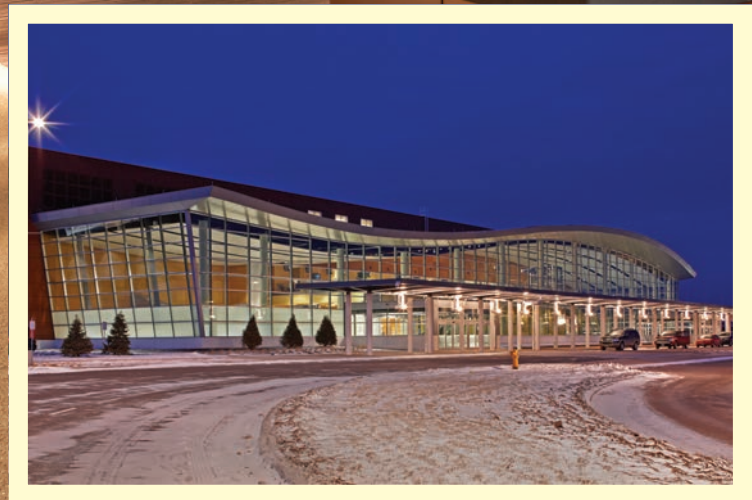
The sweeping curves of the roof line are reminiscent of the waves of Lake Superior.
