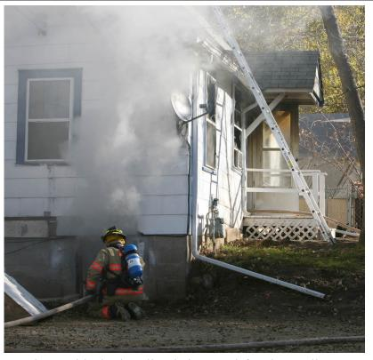
along with the hoseline being used for the appliance. This back-up or exposure line is for the protection of the firefighters. Additionally, it can be used to keep any fire from extending to the first floor.
