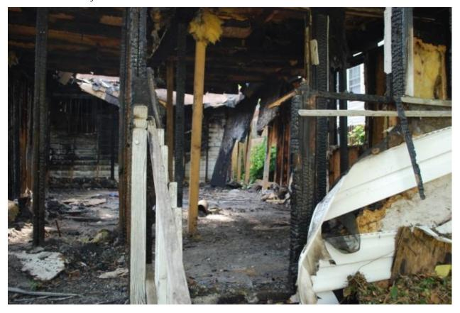
It appears that due to the substandard construction work that had been performed during construction of the rear additions, that the roof was sagging under the load and had weakened to a point of near collapse prior to the fire occurring.
