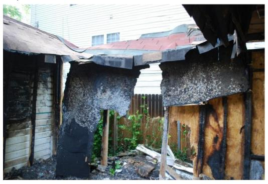
The few interior walls that were erected had a very limited load bearing capacity due to the poorly constructed floor joists and platform.
