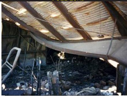
bustibles in large quantities. Don't get hung-up on the name applied to the building (fire resistive, non-combustible) because even though the building is not going to burn that aggressively, the material stored within (fire load) its contents will.
