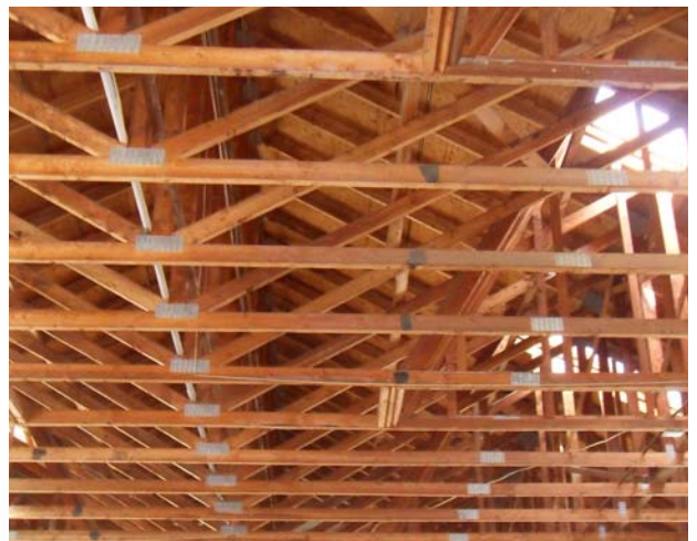
The modern fire environment consists of structures constructed of lightweight building materials capable of releasing enough heat energy to flash over a room in 7 minutes or less, causing premature structural collapse. Photo by Michael Daley
