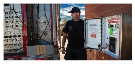
Instead of filling air bottles at the MAU, the MAU connects to the FARS external panel and piping distribution system and charges it with air. FARS are comparable to other building-installed systems, such as those used in hospitals for delivery of medical gases like oxygen. These systems are regulated under NFPA 1989, 1901, 99 and NFPA 1 as well as the International Fire Code and the Uniform Plumbing Code.
