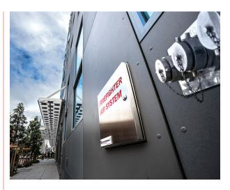
You need two things to fight a fire: water and air. Water standpipes have solved the problem of providing water inside complex structures. FARS solves the problem of air delivery.
