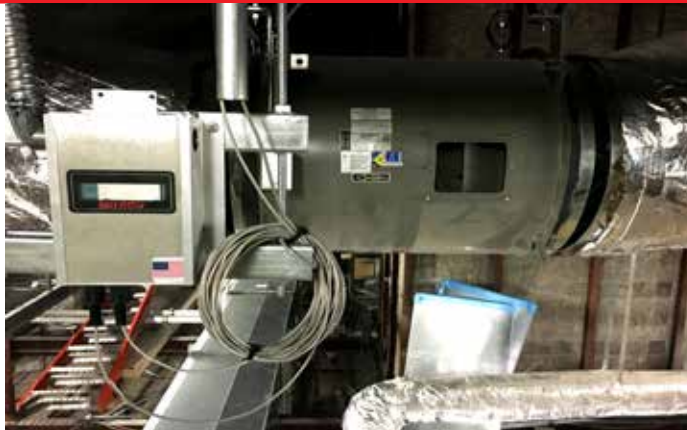
A return fan with airflow monitoring station ensures return airflow controls to the design value and will maintain the design space pressurization.
