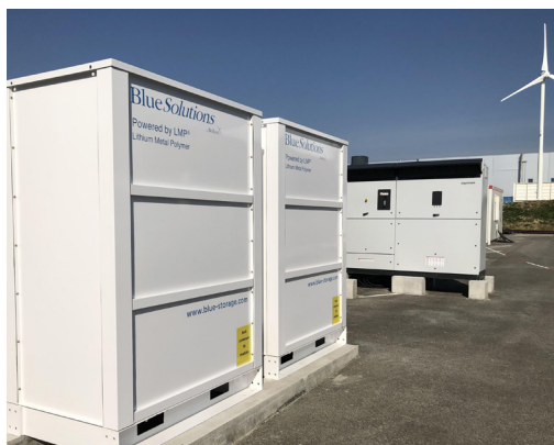
Blue Solutions batteries are solvent-, cobalt- and nickel-free and support extreme temperatures without any cooling system. Image courtesy of Blue Solutions
