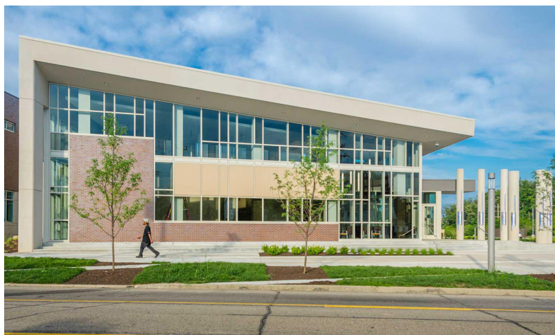
This 39,500-square-foot police station in Cincinnati achieved LBC Zero Energy Certification via a 20 percent net-positive surplus of 62,000 kwh/year that's provided to the electric grid. Image courtesy of Emersion Design
