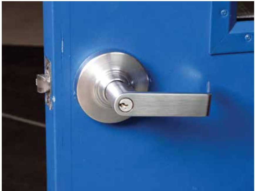
Schlage locks inside Vacaville, Calif., classrooms provide a key lock inside the classroom so the teacher can remain inside during a lockdown situation.
