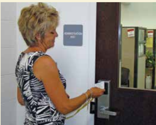
The Wi-Q system from Stanley provides access control at Stafford County schools using software, portal gateways, locksets and access controllers.
