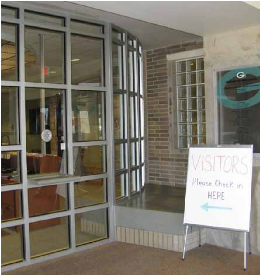
In Greenwood, Ind., a vestibule at each school routes all visitors to the office where they can be identified and screened before they are admitted. A bank teller-type window provides security while allowing for a credential exchange.
