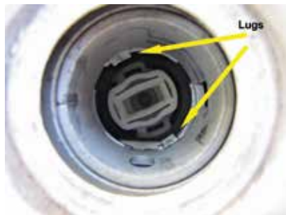
Photo 26. Lock secured into door by 2 lugs that engage in slots in lock housing.
