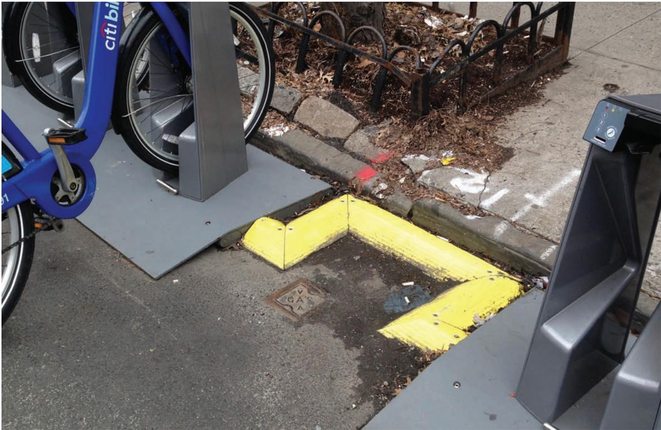
**Bridging allows the station to fit around a utility cover and provides additional flexibility in station design. Citi Bike. New York, NY**
