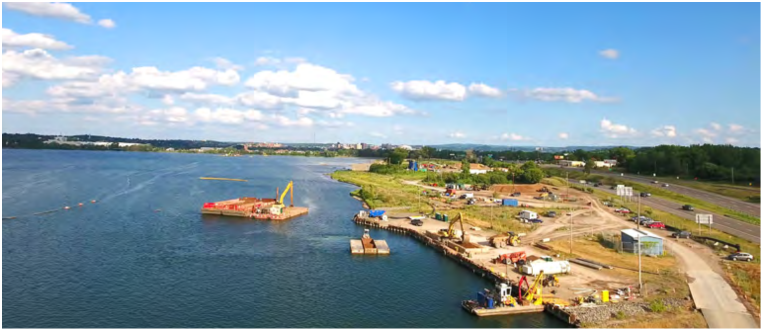
Capping equipment covering contaminated sediment with clean, stable material
