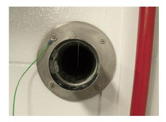
**GROUNDED DUCT** Figure 2. Ground wire was installed to prevent isolation of metal during cleaning of 4-in. duct.
