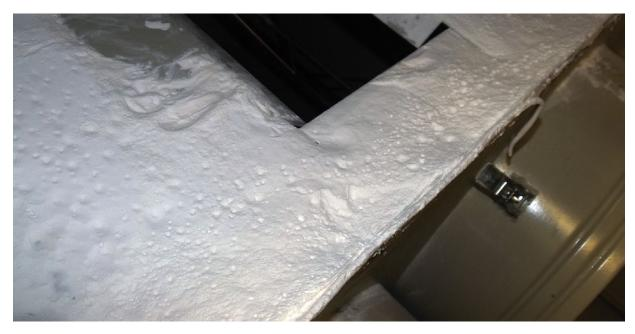
**ACCUMULATED DUST** Figure 1. Inspection revealed that interior of dust collector contained an accumulation  $\frac{1}{2}$ - to 1-in. thick.
