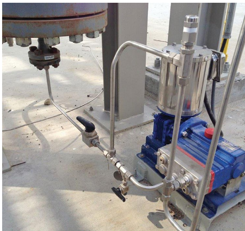
Figure 3. This seal-less pump used for chemical injection at an oil refinery replaced a pump with seals to reduce maintenance and downtime associated with seal adjustment and replacement.
