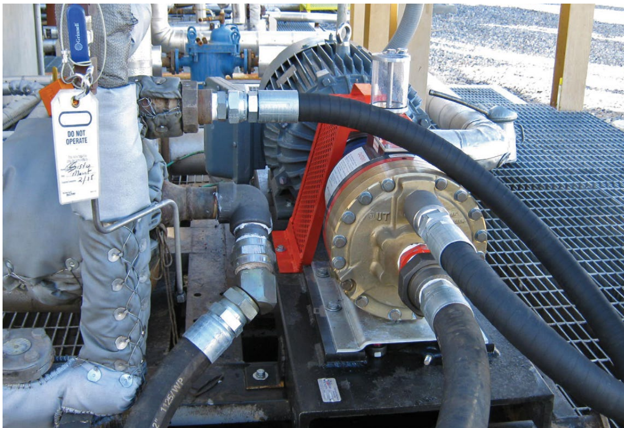
Figure 4. A seal-less pump is used for natural gas drying. The seal-less pumping chamber has no leak path, so potential emissions such as carbon dioxide are contained.
