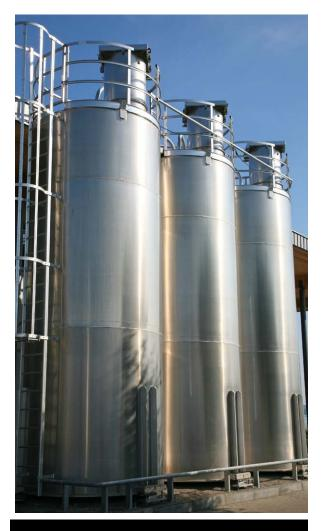
SILOS WITH WEIGH SCALES Figure 2. Weigh scales commonly are used for inventory control in silos at polyolefin plants. However, these mechanical measurements are pricey to install, replace and maintain.
