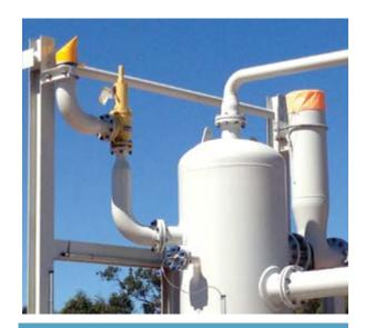
**REDUCERS** Figure 1. This piping system uses a number of concentric reducers.
