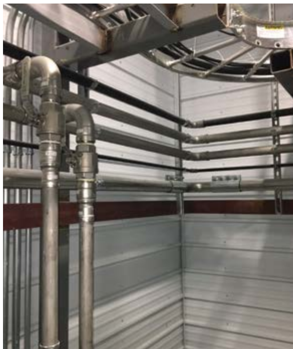
Figure 2: After other pipe joining methods caused leaks, Koppers Performance Chemicals used pressing technology to pipe a section of its facility.
