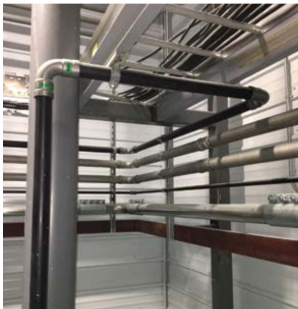
Figure 1: Koppers Performance Chemicals had 2-in. Schedule 10 stainless steel pipe installed using Viega MegaPress Stainless 90° and 45° elbows, as well as tees.
