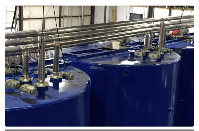
**PIPE INSTALLATION**Figure 2. Thousands of feet of pipe, with a variety of flanges, tees and 90-degree elbows, were installed over the course of four months.
