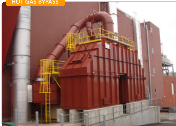
Figure 3. This RTO uses a hot gas bypass damper for high-emission loading conditions.
