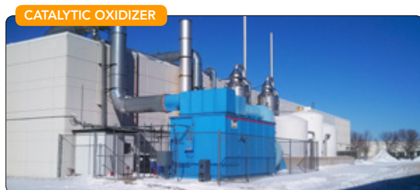
Figure 1. This catalytic oxidation system controls emissions from a batch chemical process.
