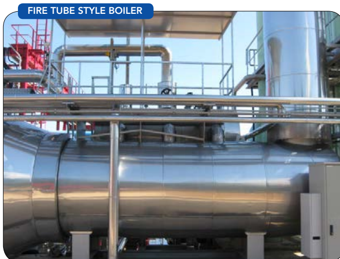
Figure 2. The system includes a fire tube, single pass waste heat boiler to generate medium pressure saturated steam.
