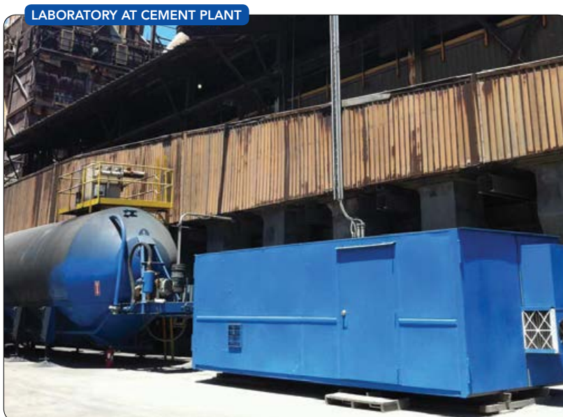
Figure 2. Vertical pipes provide laboratory (blue container) with flue gas directly from stack. Source: Oakbio.
