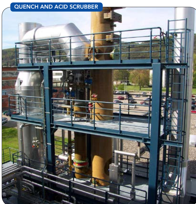
Figure 3. After exiting the economizer, the flue gas is directed to a quench and acid scrubber, much like this one.
