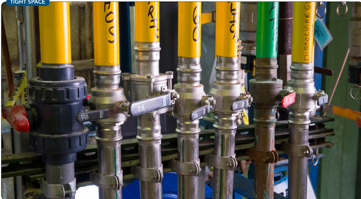
Figure 2. The pressing tool could get into smaller spaces where welding would not have been an option.
