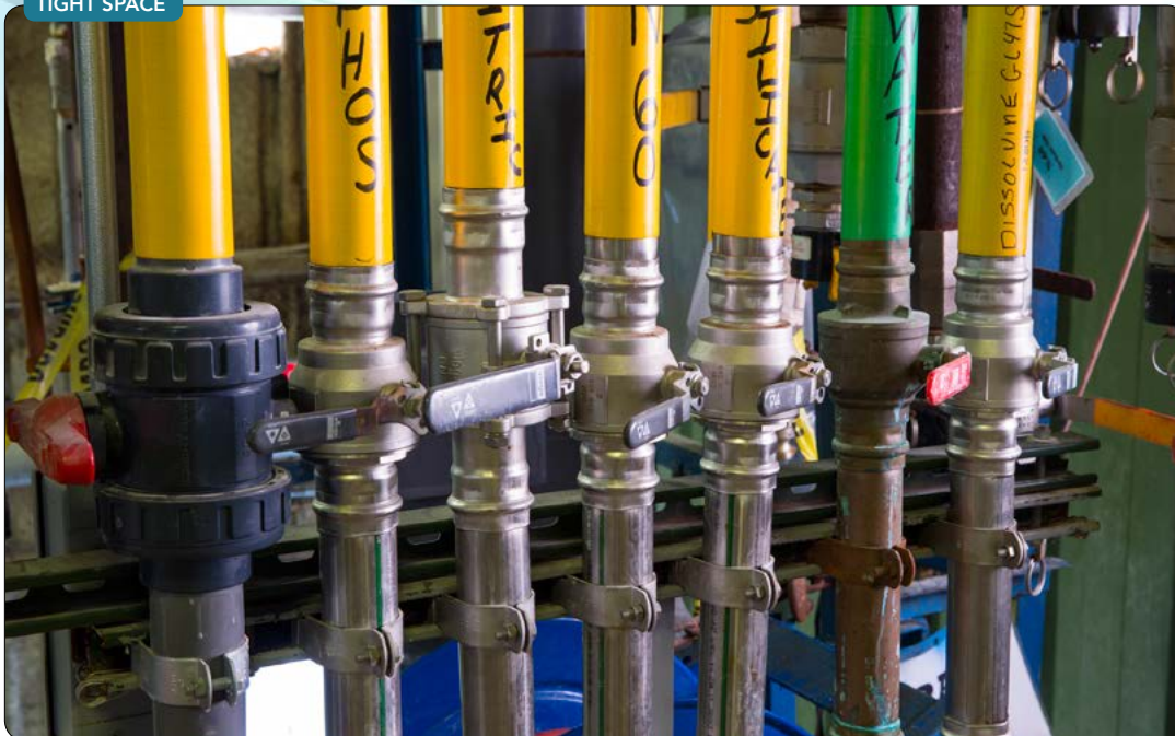
Figure 2. The pressing tool could get into smaller spaces where welding would not have been an option.
