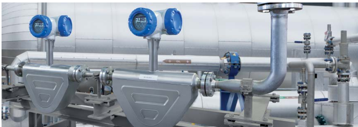
Figure 1. Newer Coriolis flow meters can more accurately detect gas entrainment and changing process conditions.
