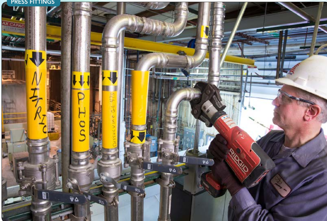
Figure 1. VIP Plumbing used press fittings to make water- and air-tight connections when adding and replacing process lines in a chemical facility.
