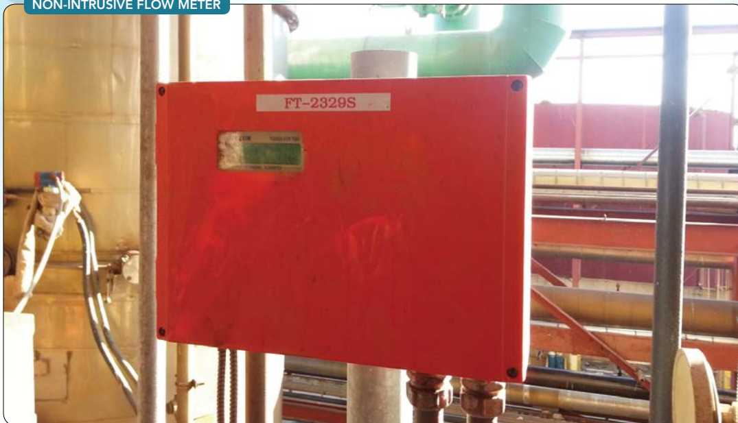
Figure 1. Because of the criticality of the flow measurement, the phenol manufacturer painted a key component of the meter red.
