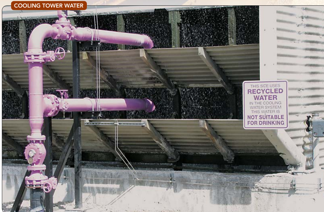
Figure 2. Facility in drought-plagued area of California has replaced potable water with recycled water in its cooling tower.
