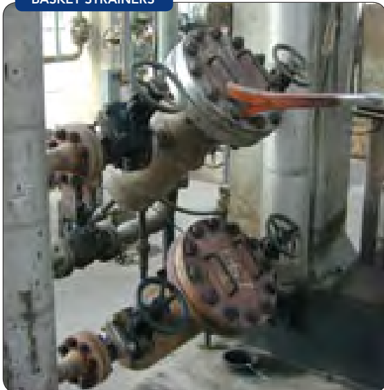
Figure 1. Permanent strainers often are installed in pairs so one always is in service.
