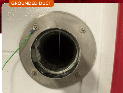
Figure 2. Ground wire was installed to prevent isolation of metal during cleaning of 4-in. duct.
