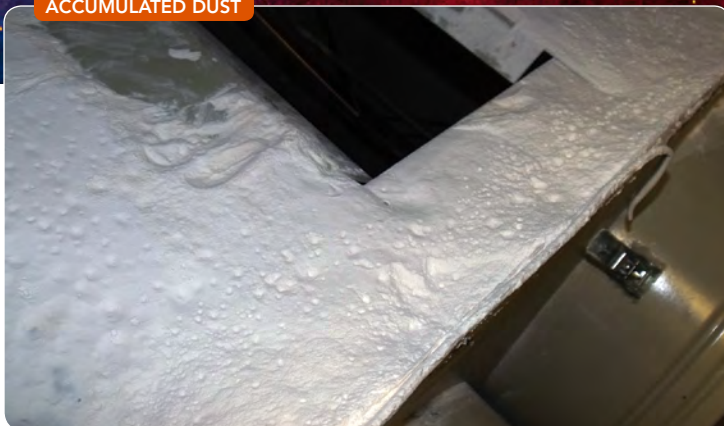
Figure 1. Inspection revealed that interior of dust collector contained an accumulation ½- to 1-in. thick.
