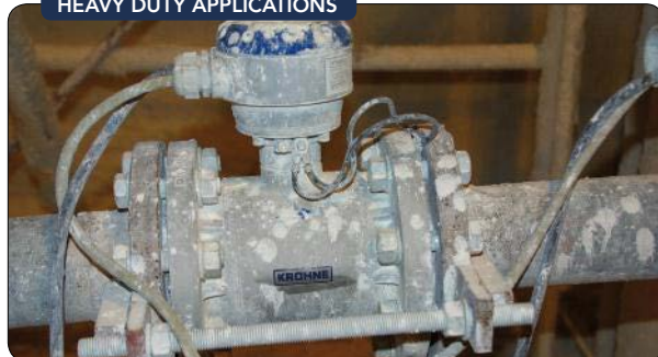
Figure 11. The OPTIFLUX 5300 measures highly abrasive magnesium hydroxide sludge.
