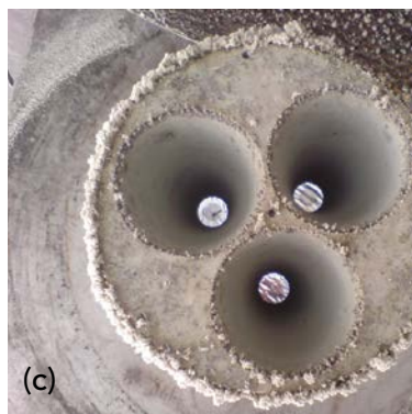
Figure 5. The scanner on a powder silo is covered with dust (a). Inside of the silo, the outside of the unit also is coated with dust (b). However, the self-cleaning sensors inside the unit are clean and fully functional (c).
