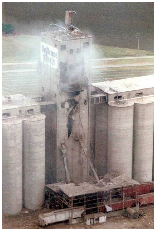
Figure 8. Dust ignited in the east tunnel of the south array of silos propagated through the entire grain elevator. Source: DeBruce Grain Elevator Explosion Report, GEEIT.
