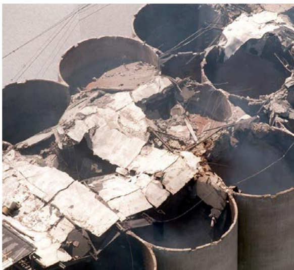
Figure 8. Dust ignited in the east tunnel of the south array of silos propagated through the entire grain elevator. Source: DeBruce Grain Elevator Explosion Report, GEEIT.
