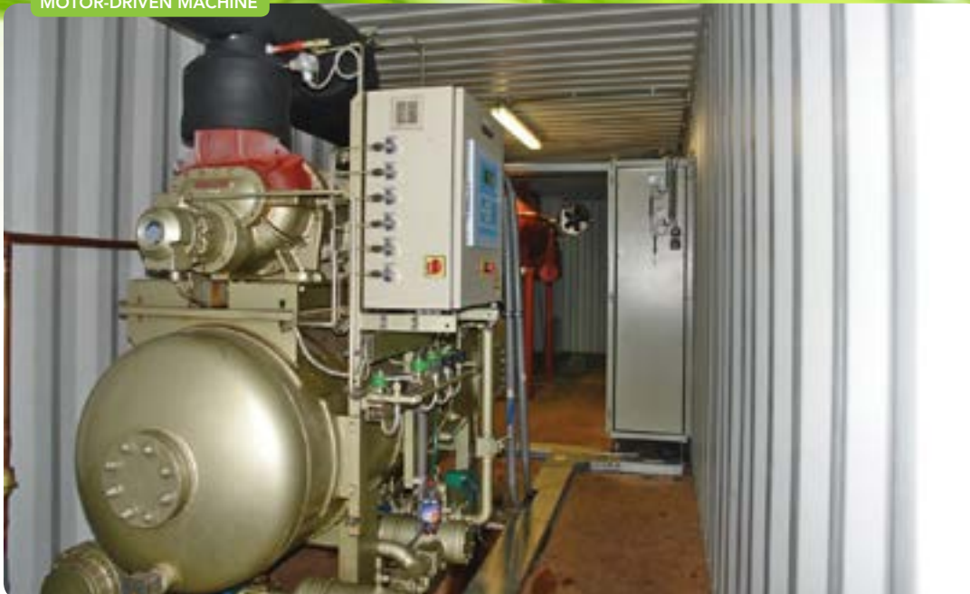
Figure 2. For small- and medium-size applications, the compressor is installed on the oil separator vessel (horizontal vessel), resulting in a compact package.
