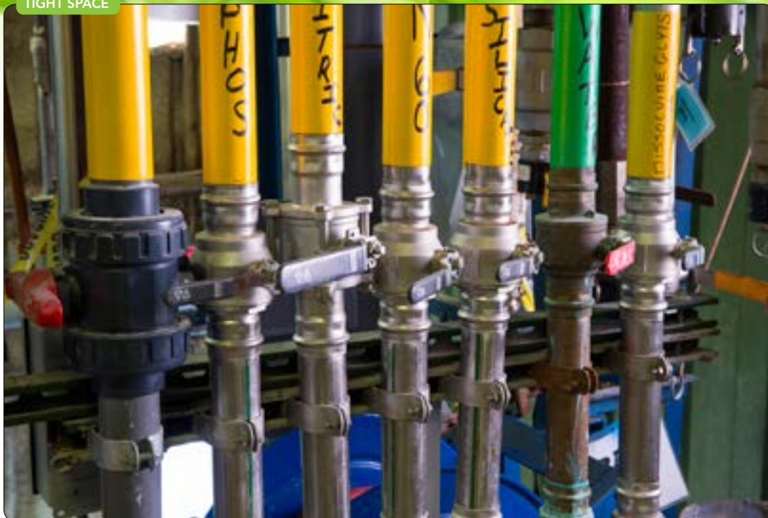
Figure 2. The pressing tool could get into smaller spaces where welding would not have been an option.
