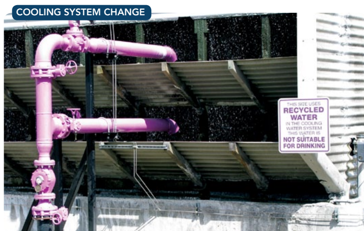
Figure 2. Santa Clara, Calif., hydrogen plant now uses recycled water as makeup for cooling system. Source: Air Products.
