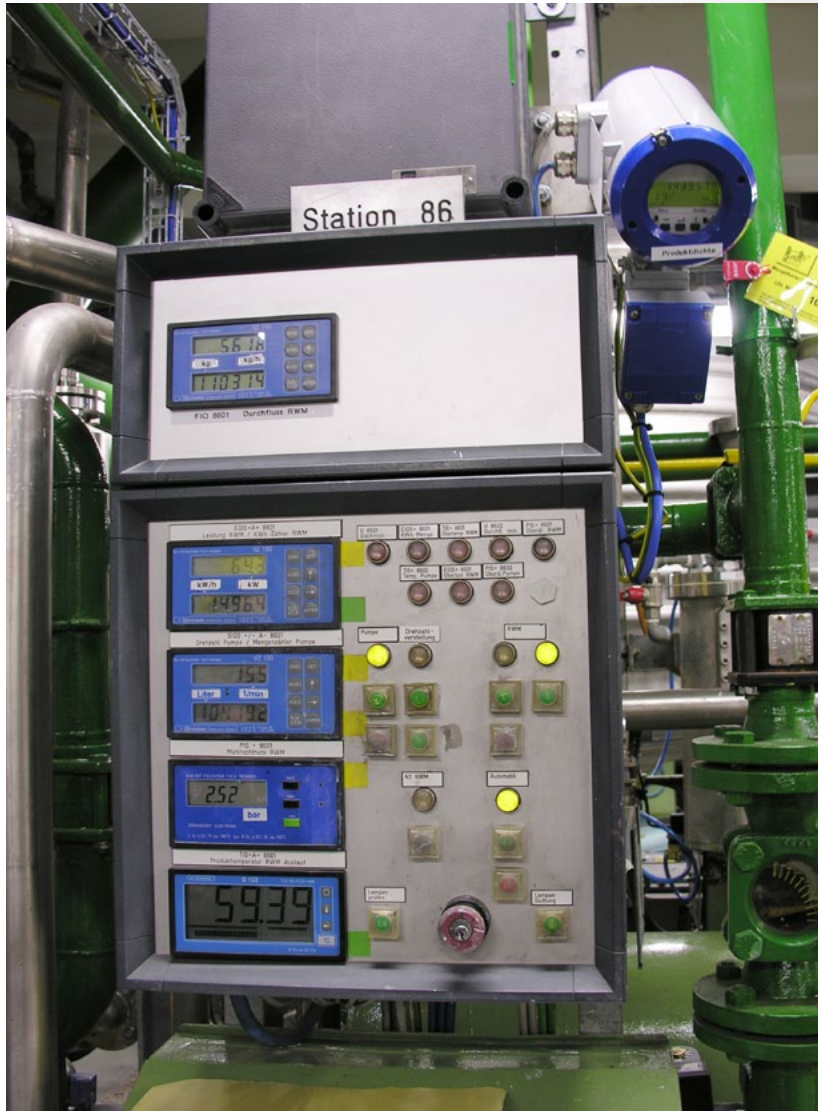
Figure 3. A programmable logic controller saves the flow measurement and compares it with the subsequent values. If there's a difference of 360kg/h, the system is automatically shut down.
