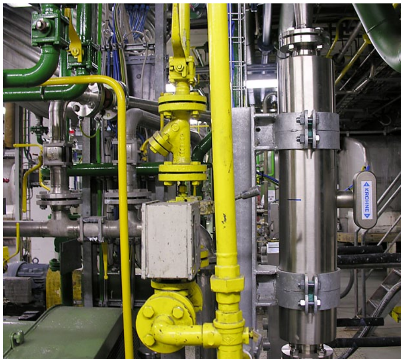
Figure 1. The OPTIMASS mass flowmeter features a straight-tube design for applications with high-viscosity media and high pigment contents.
