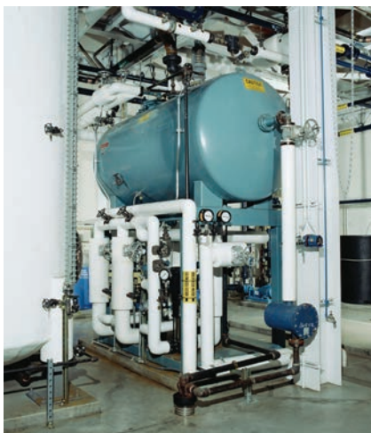
Figure 4 Deaerator (DA) tank in boiler room
