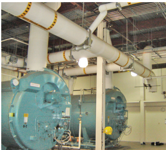
Figure 2 – Boiler header in a healthcare facility
