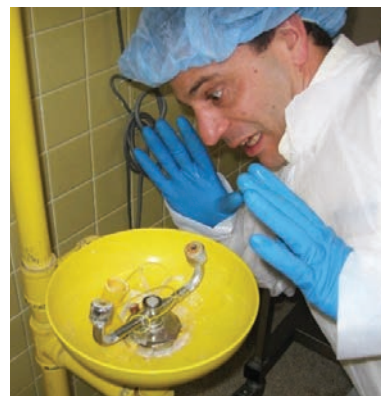
Figure 1: Eyewash with no covers on
