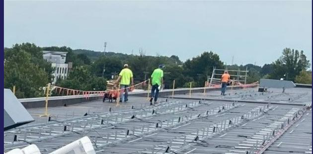
Workers are seen outside the warning line and are at the roof edge without the use of a Personal Fall Arrest (PFA) system. This type of violation is/was so severe that a work stoppage was instituted at the advisement of Edison Energy, and all personnel were retrained. Additional monitoring protocols were implemented to prevent future occurrences.
