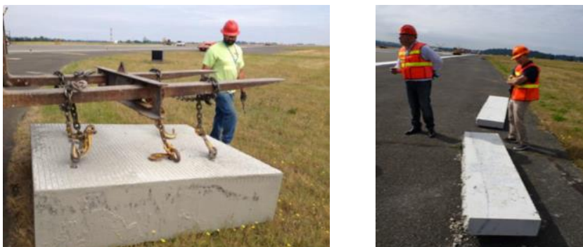
Figure 3 – Removal of Pavement After 17 Years in the Field. Runway 16R.
