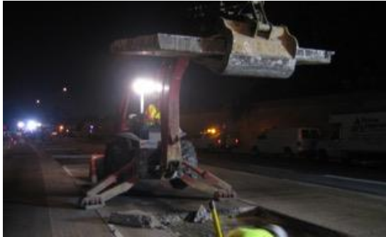
Figure 5 – ISR Removal (Left), Panel Replacement with BCSA (Right)
