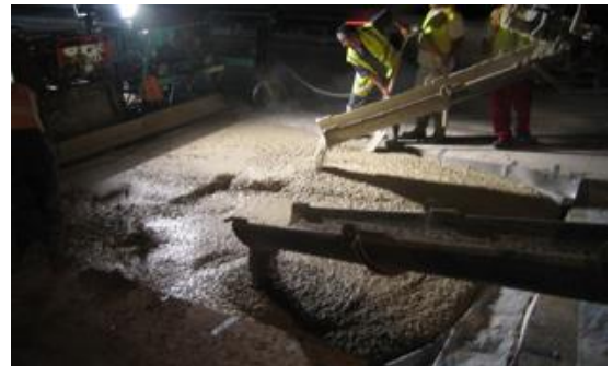
Figure 5 – ISR Removal (Left), Panel Replacement with BCSA (Right)
