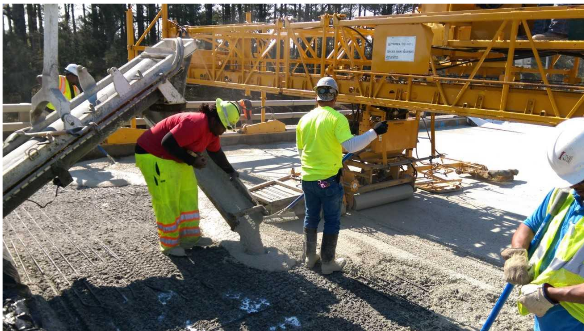
Figure 7 – Georgia DOT Rapid Set Latex Modified Concrete Bridge Overlay Project
