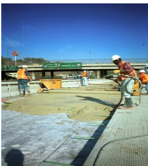
Figure 6 – JPCP Placement on I-10 (Left), CRCP Section on Highway 101 (Right)
