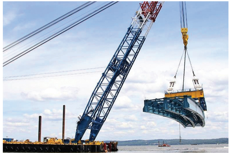
Installers assembled large sections of the bridge's structure on land before moving them into place using barges and an enormous crane.
