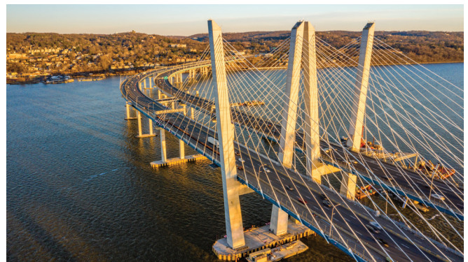
Shop applications of a three-coat system consisting of the organic zinc-rich epoxy primer Zinc Clad® III HS, an intermediate coat of Macropoxy® 646 and a topcoat of Acrolon™ 218 HS helped the Governor Mario M. Cuomo Bridge earn the SSPC 2020 Eric S. Kline Award.
