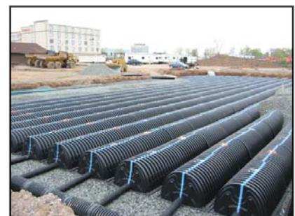
**Option #3** - External conventional pipe and fitting manifold
