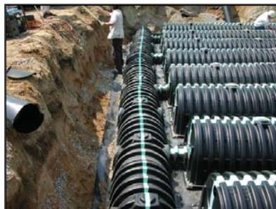
**Option #2**- External manifold using CULTEC HVLV™ 180 Header System
