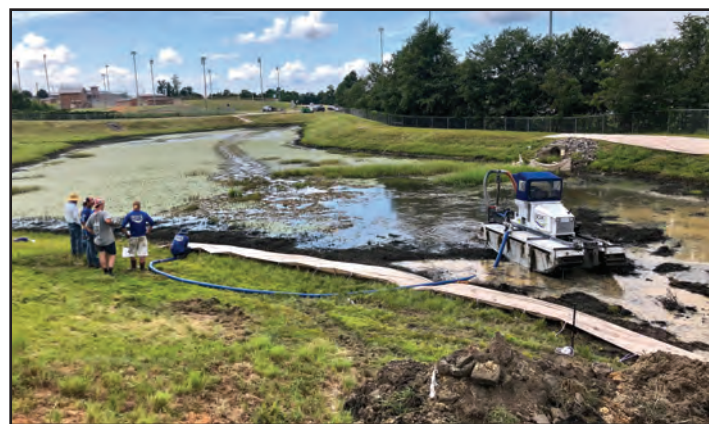
Using an amphibious work boat, pond sediment is dredged into the SOX system to stabilize the shoreline.
