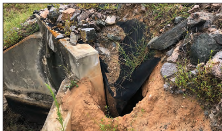
Big-box out flow culvert pipe is damaged from years of high capacity storm water run off.
