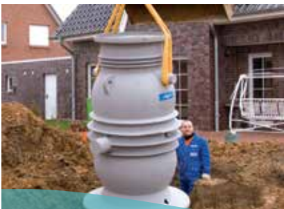
Pressure drainage plants
