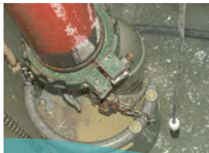
Building site pumps
