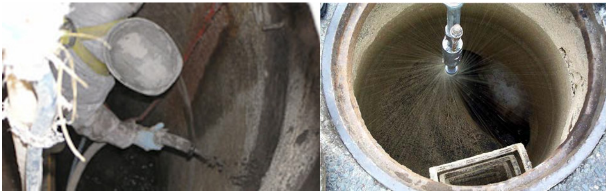
Figures 1 & 2. The figure on the left shows how the ECL is sprayed in place using a shotcrete type nozzle versus centrifugal casting in place which can deliver the ECL at a high velocity that produces good densification without the need for any troweling.
