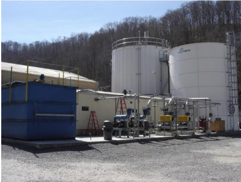
*Figure 10: AnMBR + MBR wastewater treatment system at Kellogg Company Pikeville Plant*
