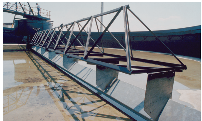
Tow-Bro® Clarifier with unitube hydraulic header for rapid sludge removal.
