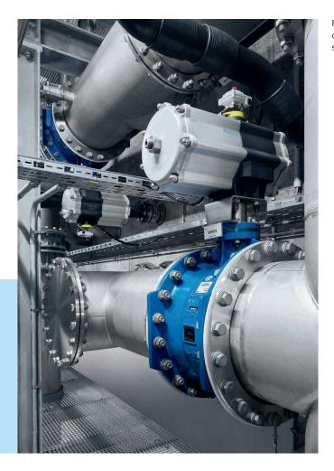
Fast, clean, safe – quarter turn actuators DAPS with de-energised normal position return to their initial state automatically in the event of a malfunction.
